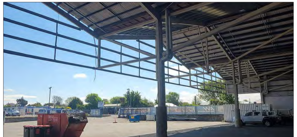
Looking out from the warehouse onsite
