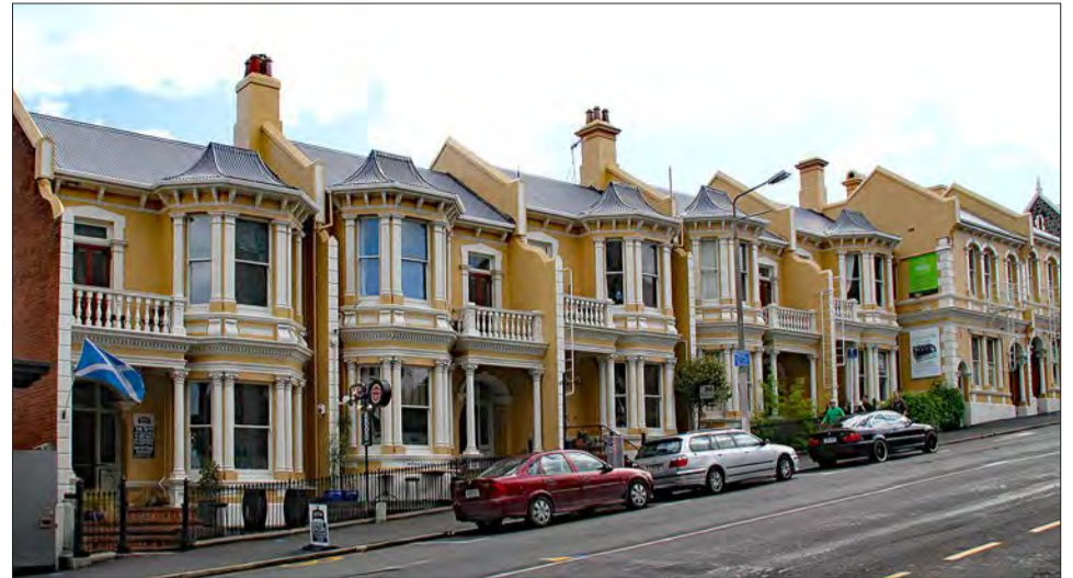
Terraced housing in Stuart Street, Dunedin (Photo: Tony Hisgett: Wikimedia Commons)
